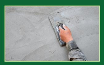
MH PLASTER RENDER 399 is a special formulated cement-sand base render contains cement, graded sand and chemicals for a wide rande of application from wall rendering to bricklaying it is prepare packed cement and sand plaster to replace the traditional on-site mixes of cement and sand.
